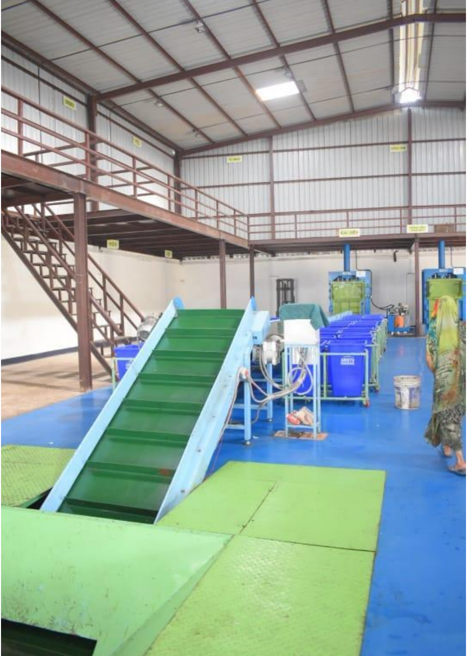
Figure 11: MRF Setup with Conveyors at Zakhira, New Delhi
